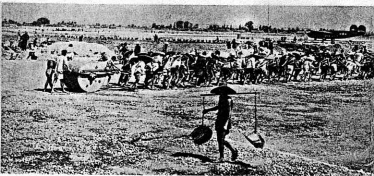
Thousands work to prepare the Superfort bases. Natives in construction crew tug on a mammoth 10-ton roller.
