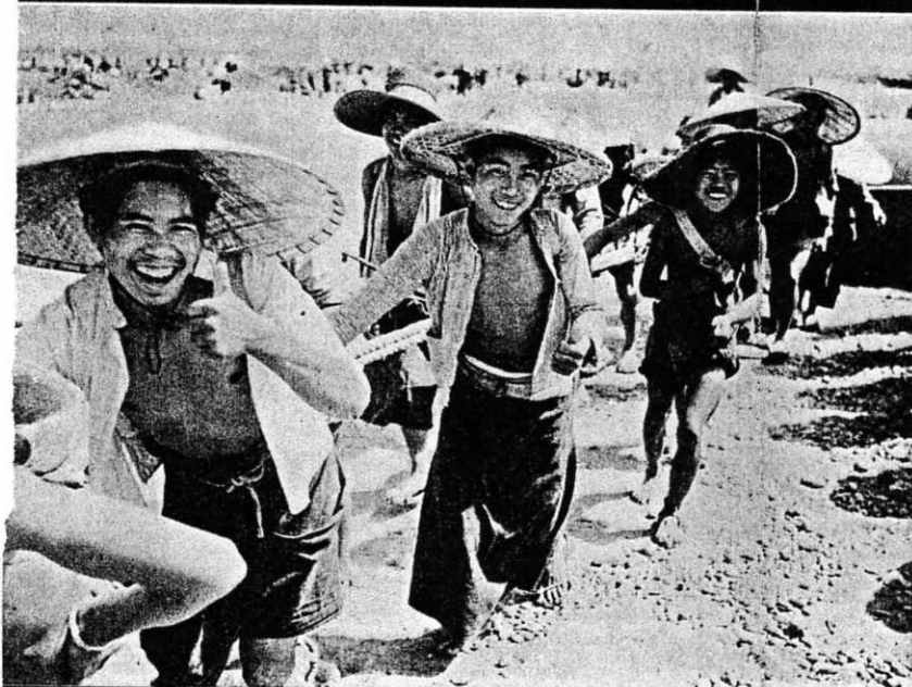
Landing strips were built by manpower. Here Chinese laborers give thumbs-up sign and shout "Ding Hao!"
